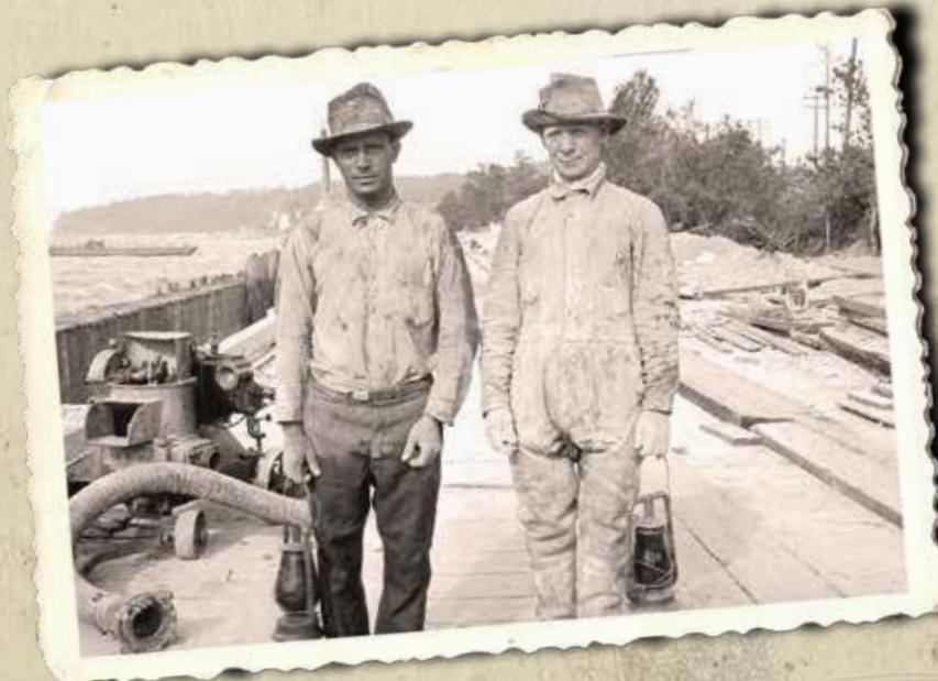
2-4 hours on a small cartridge, far longer on a large, belt-hung cartridge. If dropped, they are usually extinguished but easily relit, even if submerged in water. There is some danger from the open flame.
